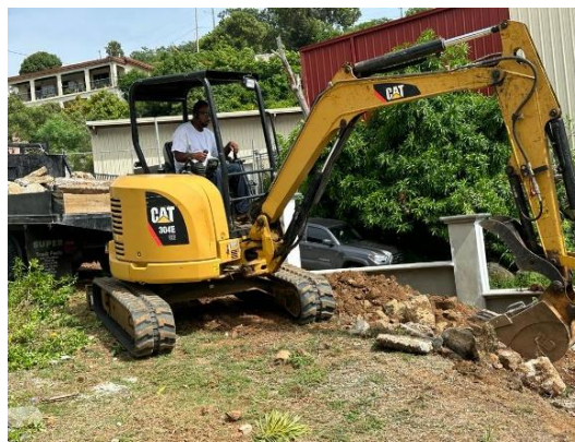
Clearing and leveling the ground around the wall
