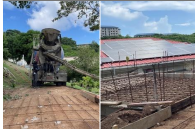
Platforms for generator and air conditioning units
