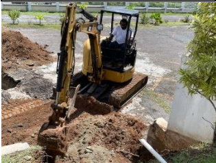
Digging for placement of pipes for electrical work
